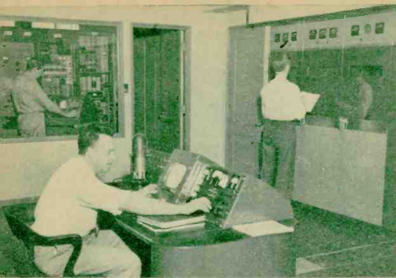
TELEVISION TRANSMITTERS, ACTUALLY MADE UP of one FM transmitter for sound and an AM transmitter for pictures, require weeks of delicate adjustment before airing. Here the engineers tune the KFI-TV transmitter before a day's beaming.
